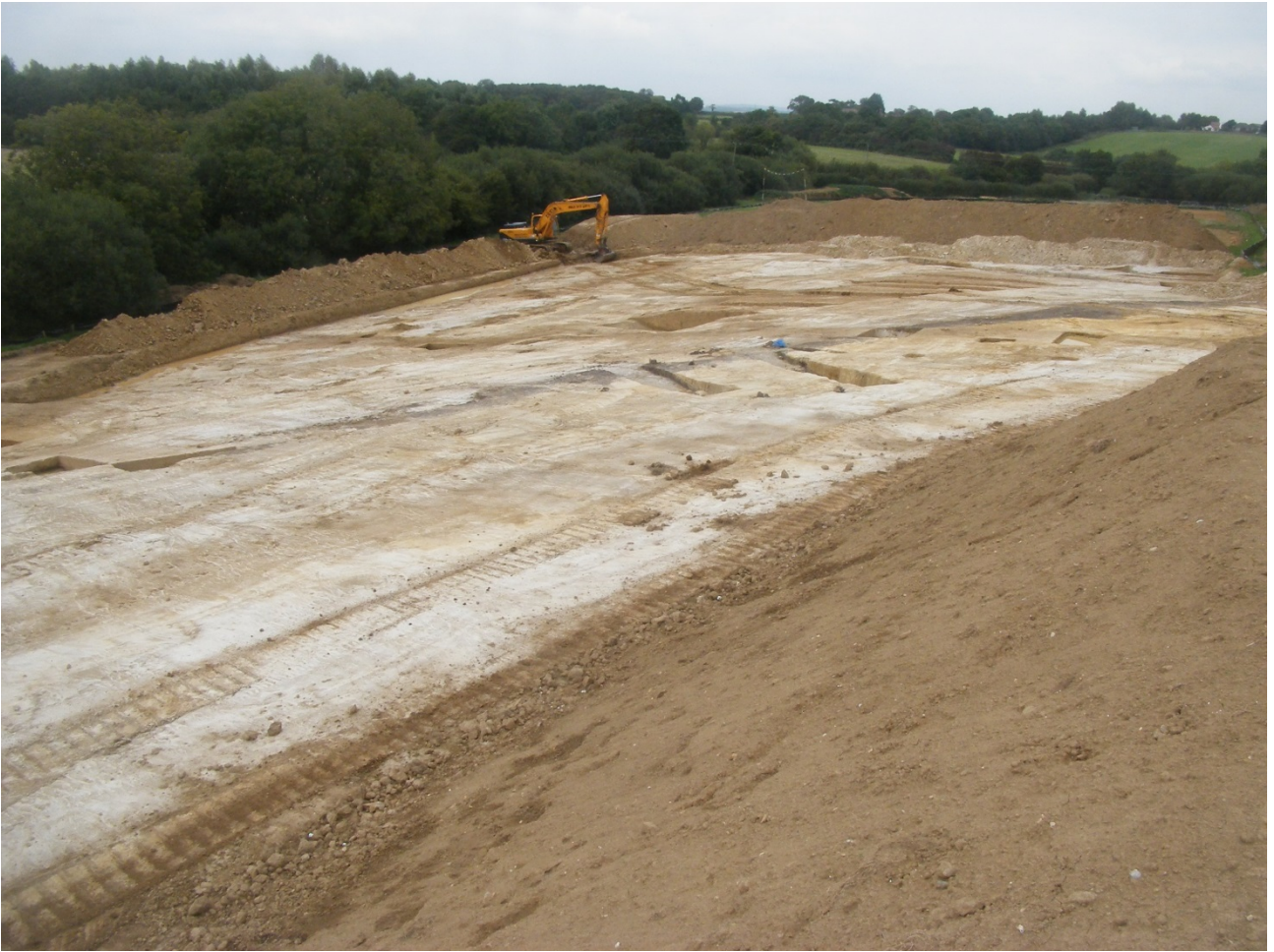
Plate 13: Area 3.2: Looking NE at the area
